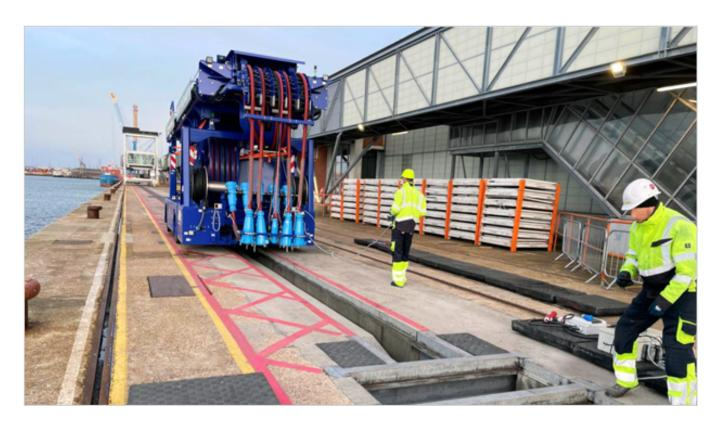
Fibrelite was approached by an OEM who provides Onshore Power Supply (OPS) systems, to quote for this large leisure cruise terminal upgrade project. The end user had previously considered Ductile Iron covers to cover the troughs housing the HV power cables and associated fixtures for their newly acquired OPS (Onshore Power Supply) system, but due to the weight of these covers and the need for specialised lifting equipment, the end user turned to Fibrelite for a solution.
