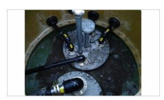
Fibrelite's vacuum testable fibreglass tank sumps and 25 ton rated GRP composite covers are being installed in both Norway and Finland.
