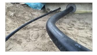
An important component of this system is the innovative and efficient corrugated pipe system FLEXWELL® All-in-One for the transportation of liquefied natural gas from the storage tank to the pump.
