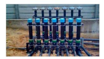
All **SMARTFLEX** primary piping consists of a multilayer composite wall lined product pipe that combines the excellent mechanical properties of HDPE with the low permeability and high resistance to hydro-carbons of a new class of polymers used in the lining material and creates a level of hydro-carbon compatibility unattainable by other fuel pipes available on the market today.
