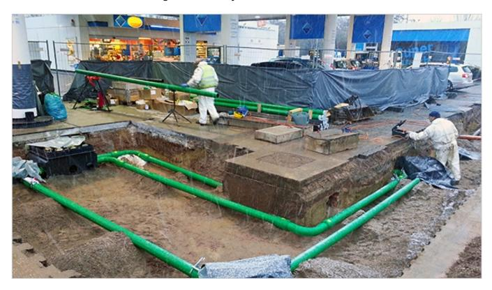
This case study tells the story of a project completed before the lockdown went into place, where KPS worked with BP Aral in Germany (Gotha) to replace their previously installed metal pipework with our corrosion-free double wall polyethylene piping, protecting people and the environment.
