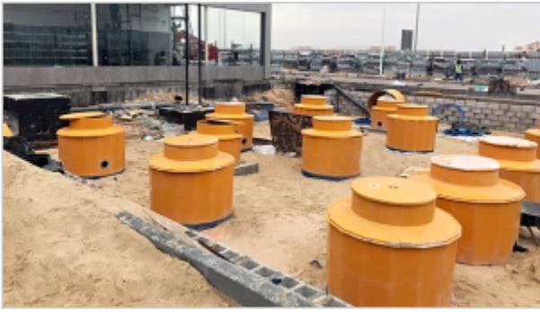
Vacuum testable Fibrelite GRP sumps provide a strong, durable, liquid-tight containment solution | © OPW Global
