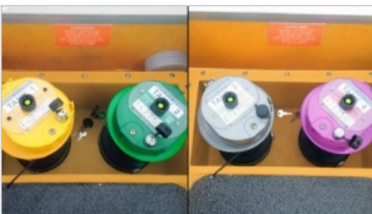
The fully conductive below ground remote fill systems are supplied with a non-slip working platform for the tanker driver to stand on. // Factory fitted with dual contained KPS pipework for fills and single wall for stage 1 vapour line.
