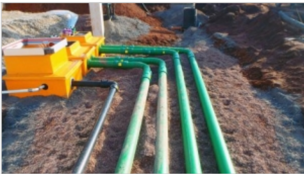
All integrated KPS fittings weld both pipe walls simultaneously
