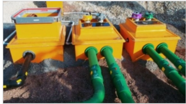
Fibrelite's below ground remote fill systems with factory fitted/tested dual contained and conductive KPS pipework
