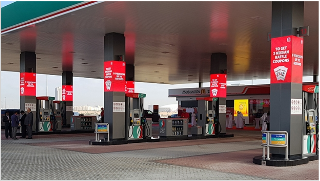
Digital screens at an ENOC station
