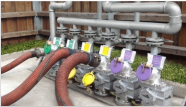
MIDAS from Berrys ensures misfuel/crossover prevention in all conditions.
